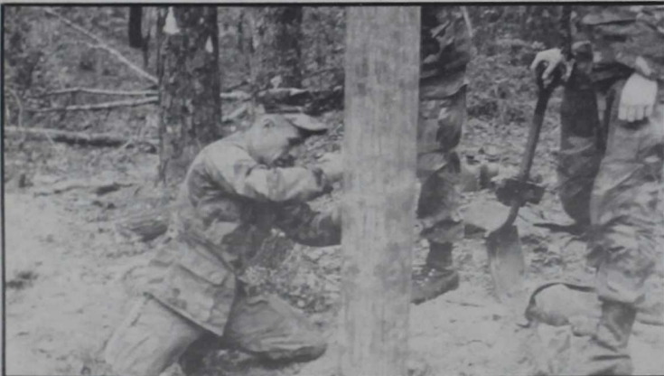
Lance Cpl. David C. Randle, Charlie Co., 8th Eng. Sup. Bn., 2nd FSSG, secures the pole to the "Tarzan Swing" by pounding the dirt firmly around it.
