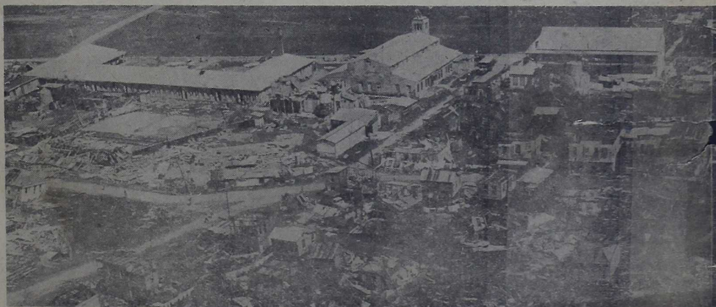
DEVASTATION — This is the city of Stann Creek in British Honduras after Hurricane Hattie raised havoc with the town of 8,000. Some 250 died in this sn... only buildings left
