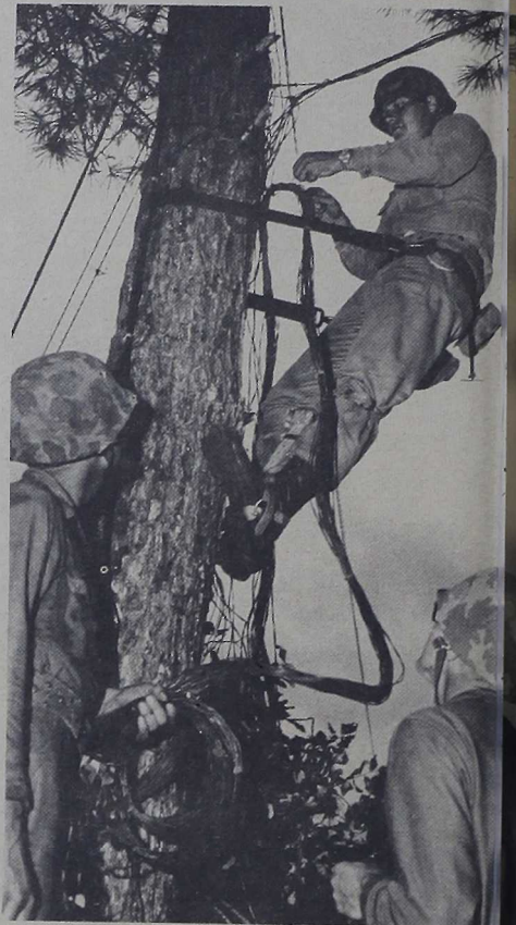
INSTANT TELEPHONE POLES —Corporal Richard W. Fleischer, Jr., Communications Company, Headquarters Battalion installs telephone wires during 2d Marine Division Command Post Exercise. (Photo by Sgt. R. E. Priseler.)
