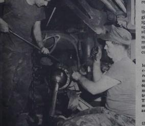
AXLE REPAIR — Marine Lance Corporal James Wood, left, and Private First Class Roy Stiftera work together while repairing an axle in the heavy equipment section of the Marine Force Logistic Command's Engineer Maintenance Company.
