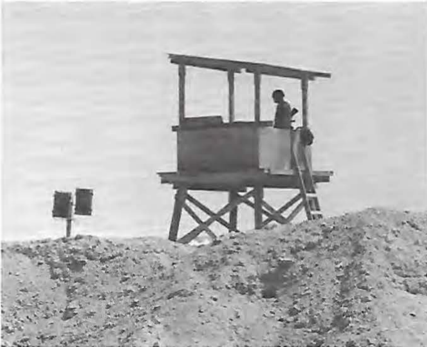
Guard tower with earth berms to protect against indirect fire.
