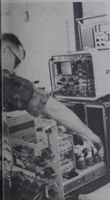
Missile maintenance technician, Sgt. Jeffery Prickett, ensures the serviceability of a Dragon missile set before beginning a calibration test.
