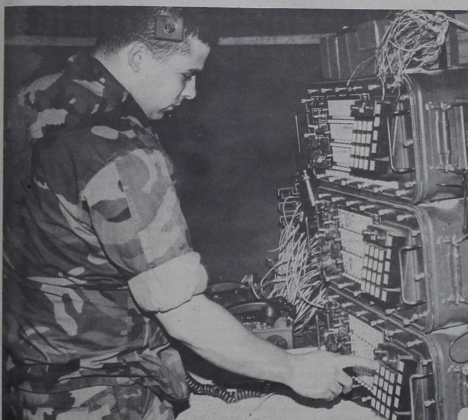
Sergeant Carlos R. Rodriguez, wire chief, patches a call through on the backup switchboard.
