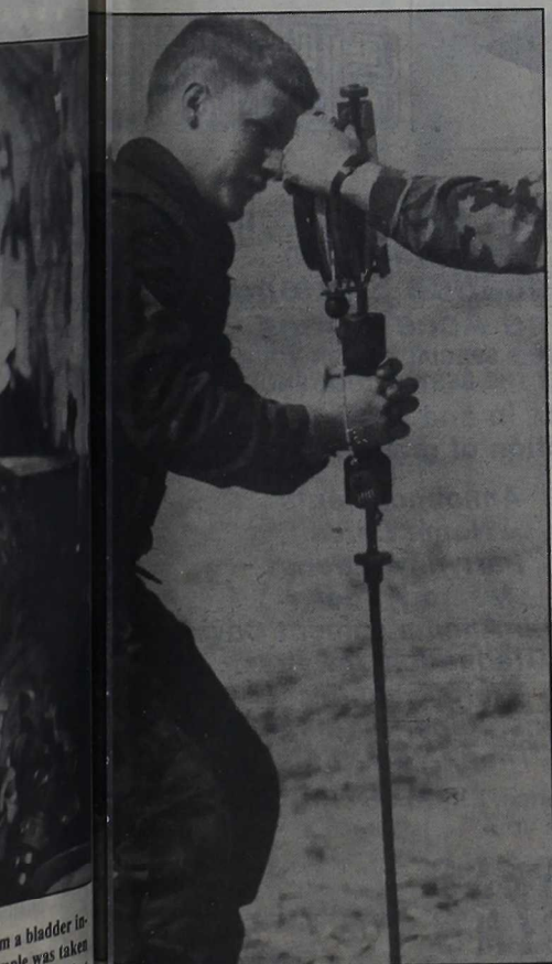
HMM-263, 24th MAU, pounds a grounding stake as part of the setting up of a Forward Arming and Refueling Point (FARP). The FARP was part of a long range raid exercise. (Photo by GySgt. J. Booker Simmons)
