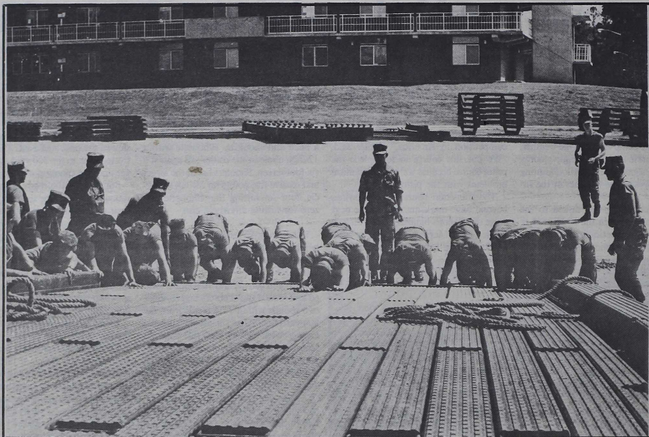
ANCHORS AWEIGH — Engineer students give the 24-ton, 92-by-44 foot floating bridge a little help getting off the shore.
