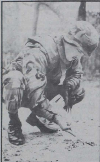
PROBING — A Marine from Bravo Co., 8th Engineer Support Bn., probes for a possible mine after a mine sweeper picked up a tone in that area.
