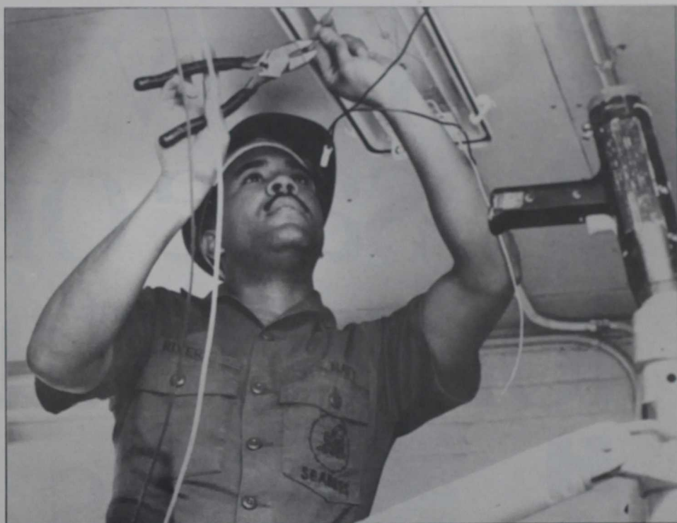
CE3 Darryl A. Rivers rewires the lighting throughout the buildings.
