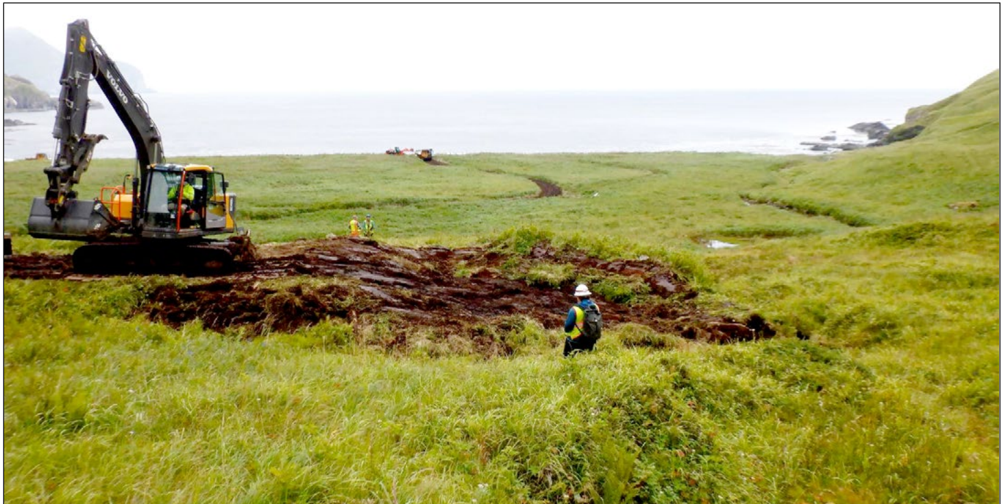
Crews work to recontour excavated areas to match the surrounding topography and replace the organic layer at the Cape Prominence Formerly Used Defense Site.
