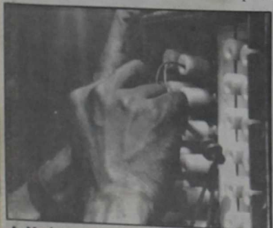
A Marine connects telephone wires to a terminal box during a division exercise.
