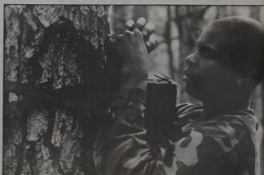
Sgt Willie E. Covington, Communications Company, Headquarters Battalion, connects telephone wires to a terminal box attached to a tree.
