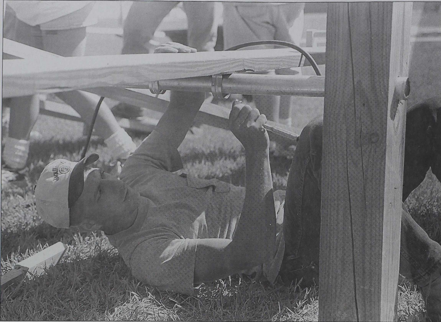
Cpl. Joe A. Fisher applies brackets to a see-saw to maintain safety and stability.
