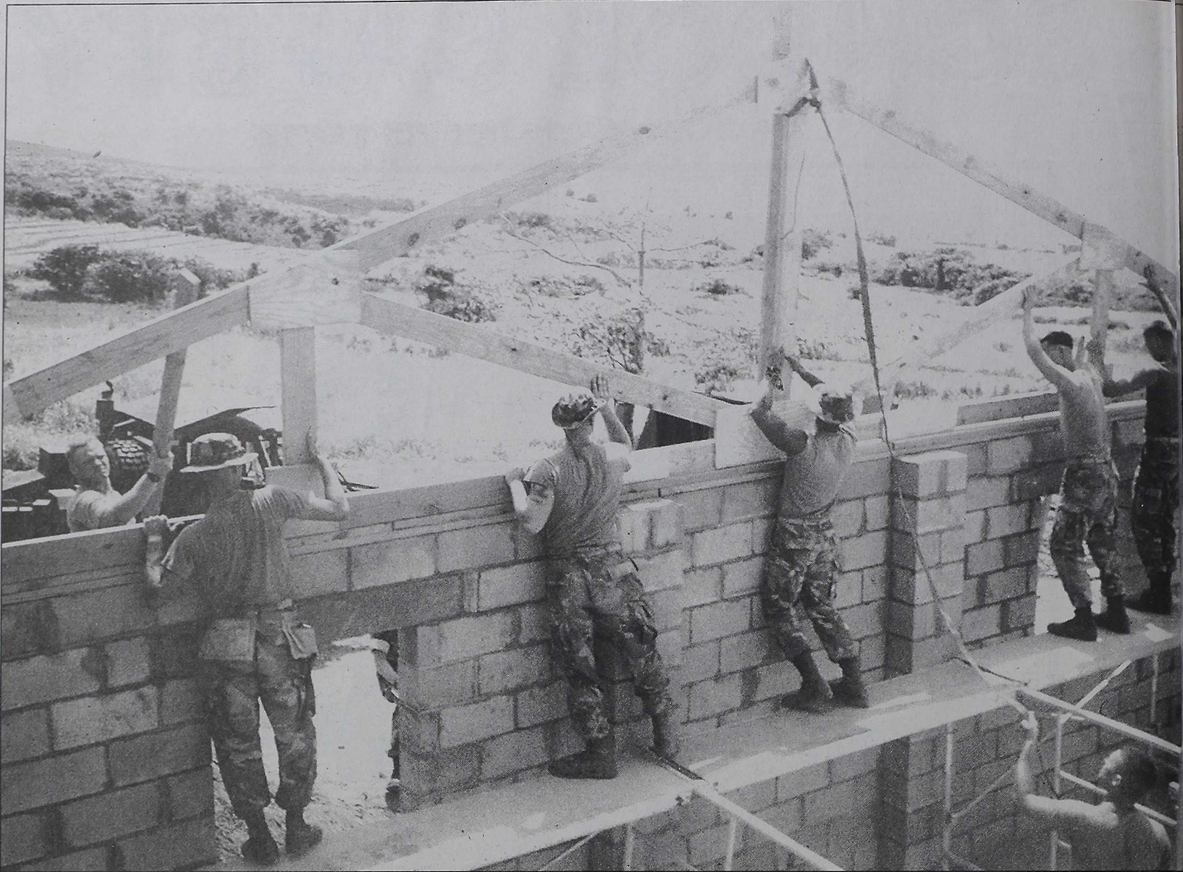
Combat Engineers lift and secure an "A" frame to a building.
