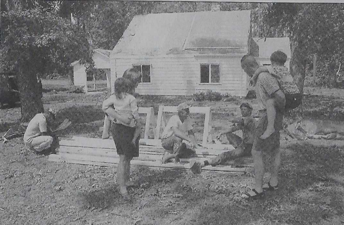
Above: The Gards talk to rebuilding crews about the extent of the damage to their home. (Photo by Cpl. J. J. Rodriguez) Right: 1stLt. Brian Gard stands next to the area where the second tree hit his house, causing a metal beam to nick him in the forehead. (Photo by Cpl. J. J. Rodriguez)
