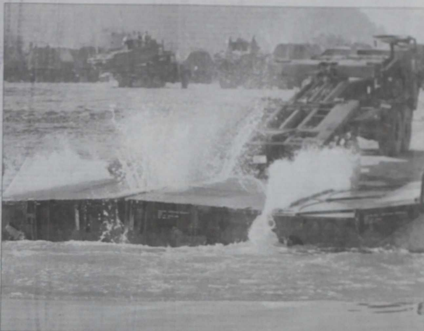
An interior bay blooms open after being launched from a logistics vehicle system on the Han River Nov. 1. Service members from 9th Engineer Support Battalion, 3rd Marine Logistics Group combined efforts to assemble a portable, pontoon bridge over the Han River at the Haeng Ju Bridge Training Site Oct. 27 through Nov. 2.
