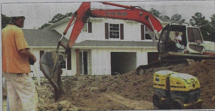
Dave Phillips, a pipe layer with South Side Utilities in Jacksonville, operates a roll ramp while Brian Hoffman, a track hoe operator with SSU, moves dirt at one of the new housing construction sites on Tarawa Terrace I, July 12.
