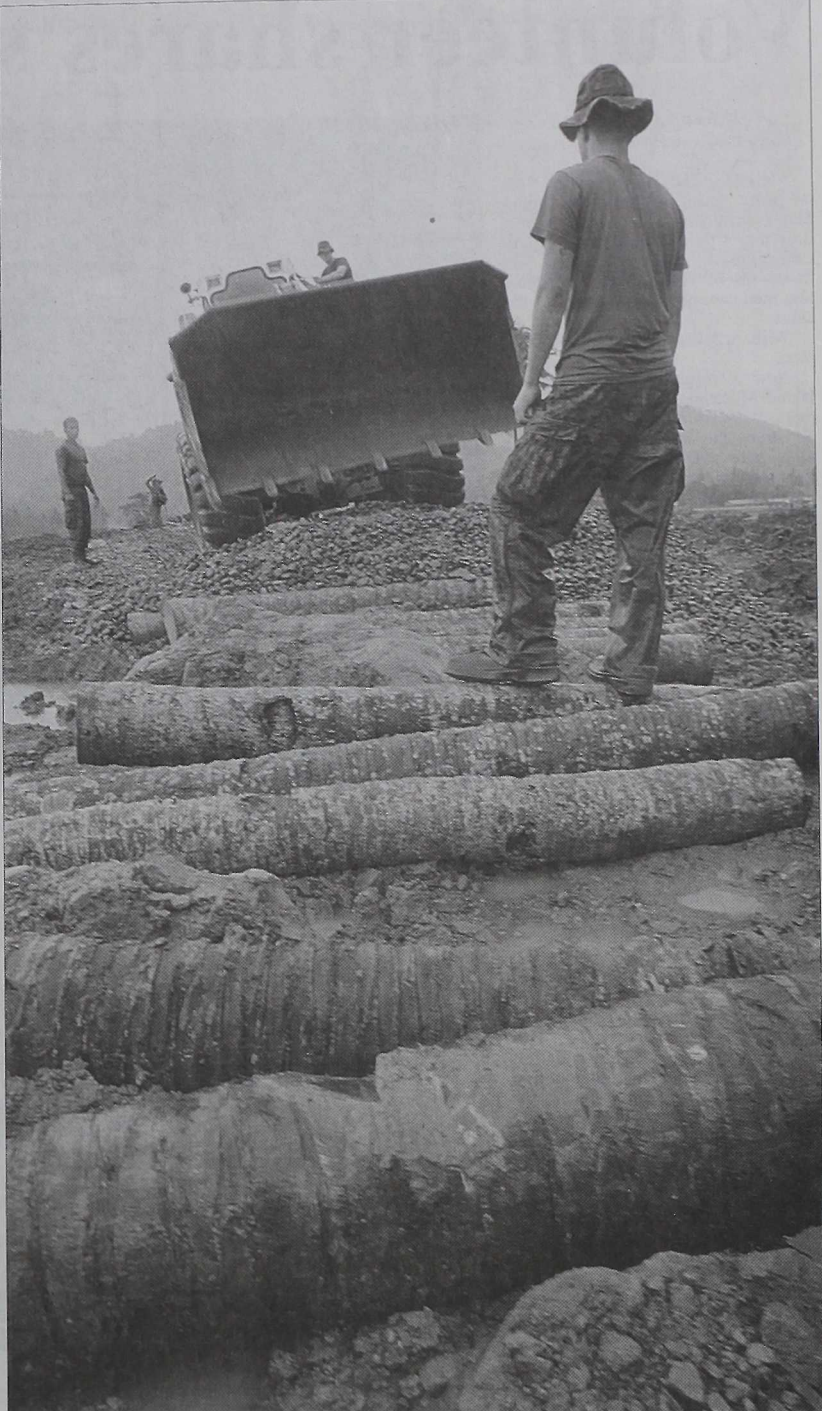
Cpl. Martin R. Harris Southern Leyte, Philippines: Marines with combat engineers detachment, 31st Marine Expeditionary Unit, are using logs cut from nearby trees as foundation for a road they are building to the landslide disaster area in Southern Leyte, Philippines.
