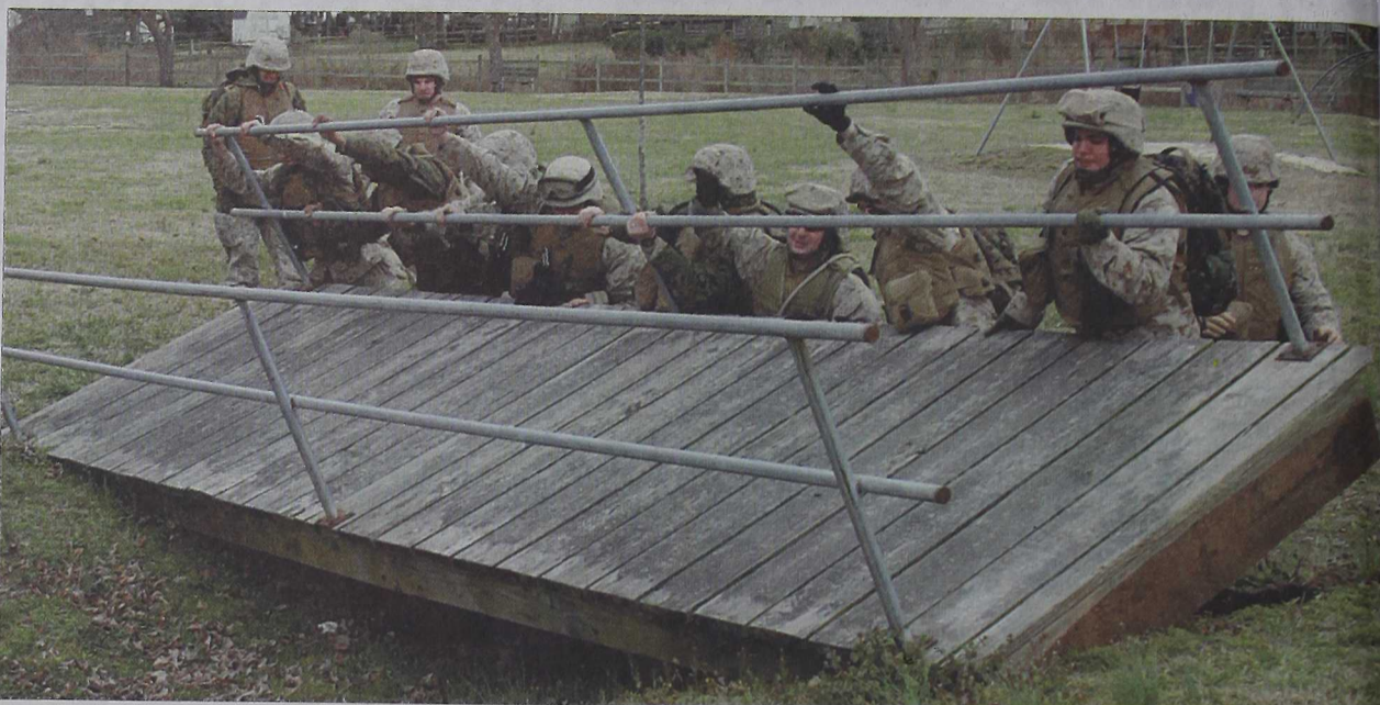
Virginia Beach, Va.: Combat engineers attached to the 24th Marine Expeditionary Unit, tear down two bridges at Salem Woods Residential Park in an Urban Environment Exercise.
