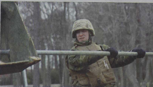
Virginia Beach, Va.: Gunnery Sgt. Carl Zador, a combat engineer with MSSG-24, breaks a metal hand rail that used to be attached to an old foot bridge at Salem Woods Residential Park.
