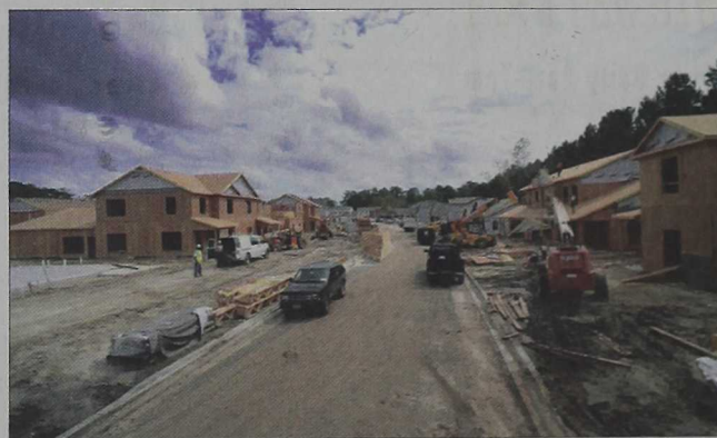
The new construction at Tarawa Terrace is moving forward at a rapid pace. Photo by Ena Sellers
