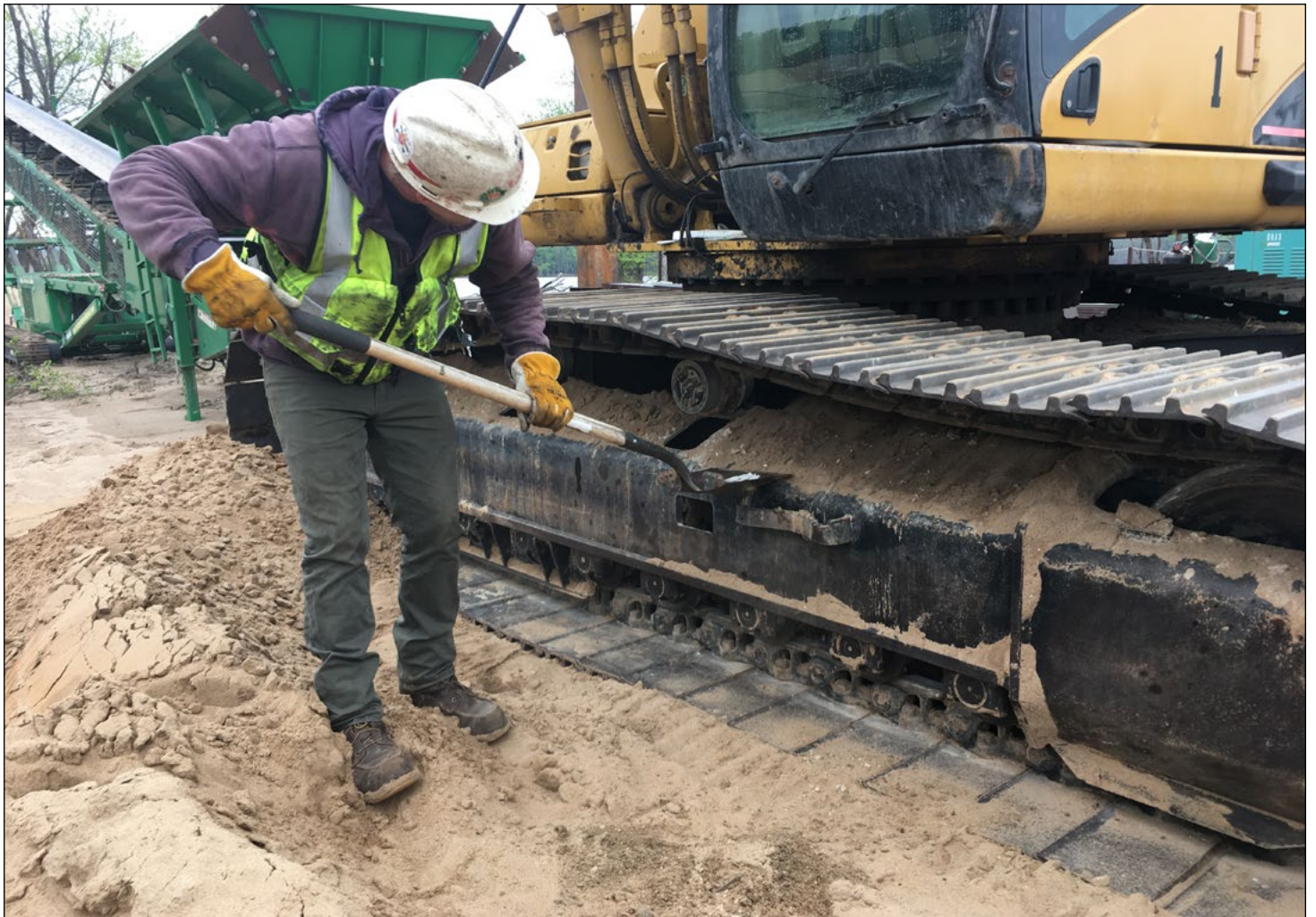
Scott Rolbiecki, master tender operator, USACE, St. Paul District, removes sand from the tracks of an excavator before dredged material placement at McGregor Lake near Guttenberg, Iowa, May 21.
