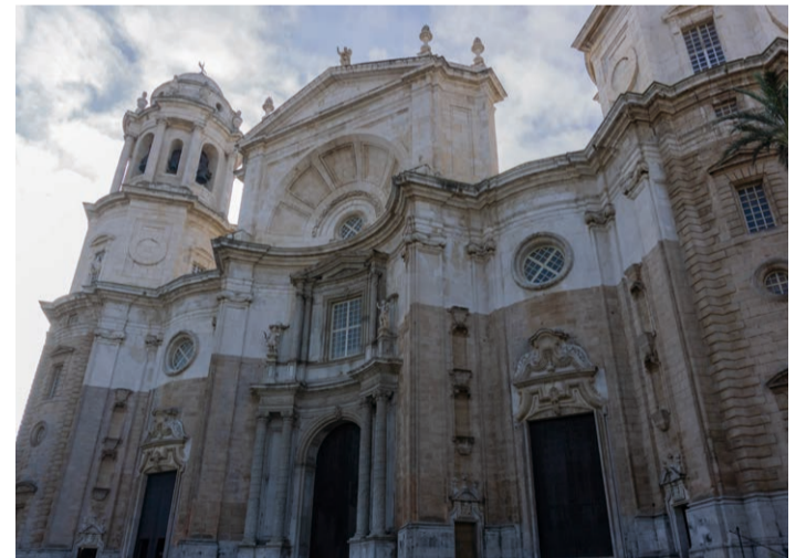
A trip to Cadiz should include a stop at the Cadiz cathedral. An interesting note is that during the construction of Catedral de Cadiz the building materials were changed three times due to financial instability. The changes in stone are clearly visible, and give the cathedral a distinct look.
