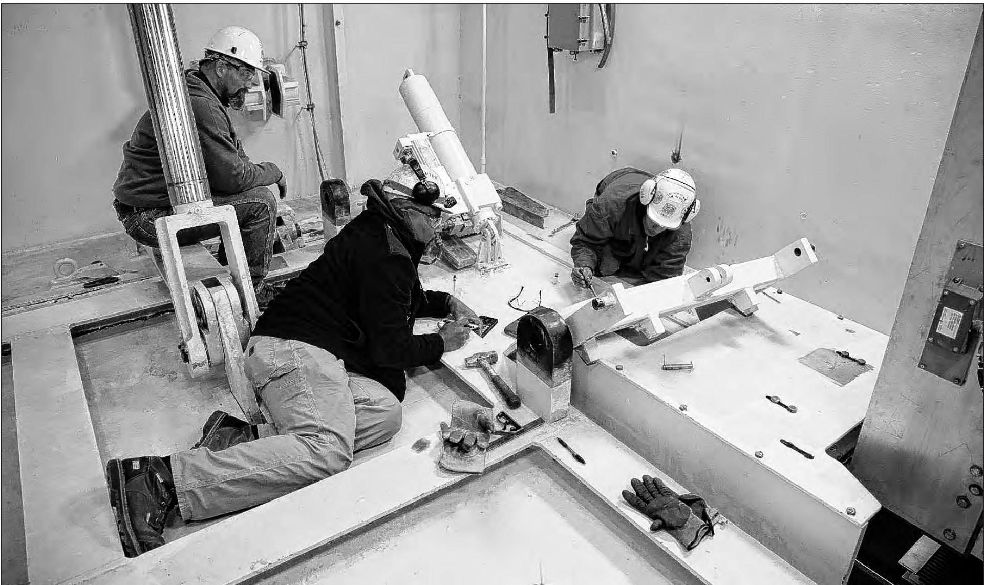
MCSA Riley McDowell Huntington Ingalls Industries-Newport News Shipbuilding Division contractors aboard the aircraft carrier USS Gerald R. Ford (CVN 78) conduct phase 2 testing on a lower stage weapons elevator. This testing marks another milestone in the certification of Gerald R. Ford's Advanced Weapons Elevators.
