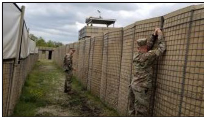
Soldiers attaching the FlexZone to a facility perimeter
