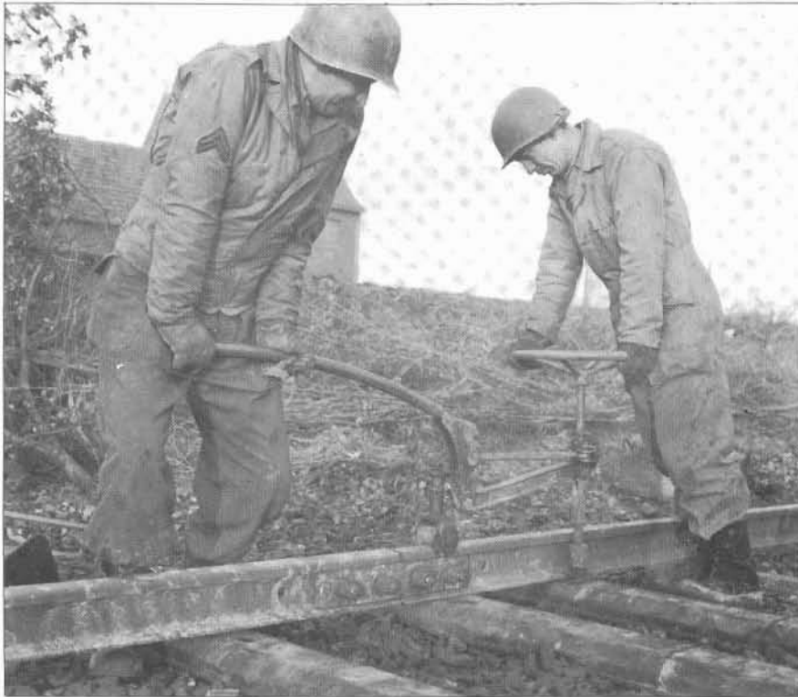
Captured German equipment is used by engineers of D Co., 332d Engineer Reg., to repair a railroad near Aldenhoven, Germany, during World War II.
