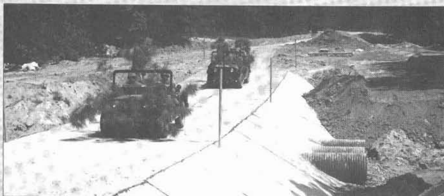
Low-water crossings make swampy areas at Ft. Polk passable at all times.
