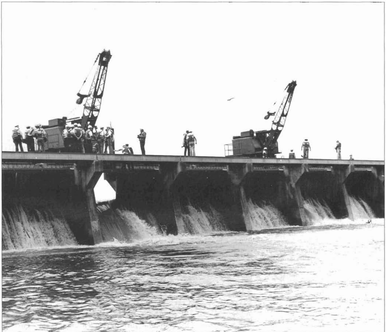
Water pours through one of Bonnet Carre's 350 bays. (U.S. Army photo.)
