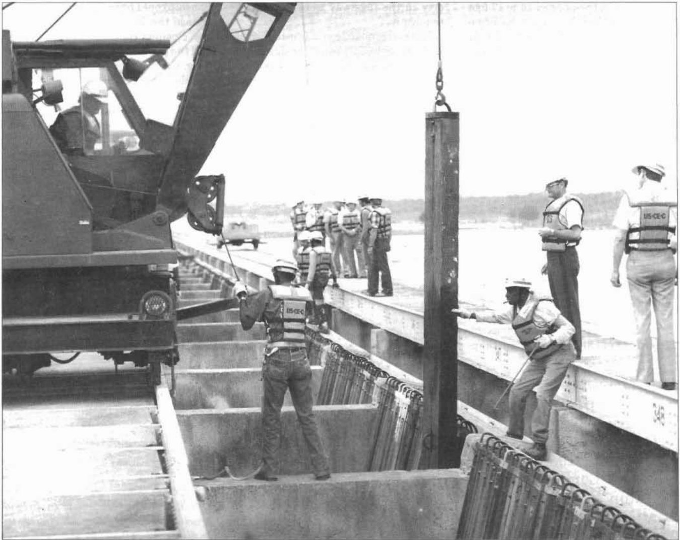
A crane atop Bonnet Carre Spillway pulls an 8 x 11½-inch timber "needle" from a bay. (U.S. Army photo.)
