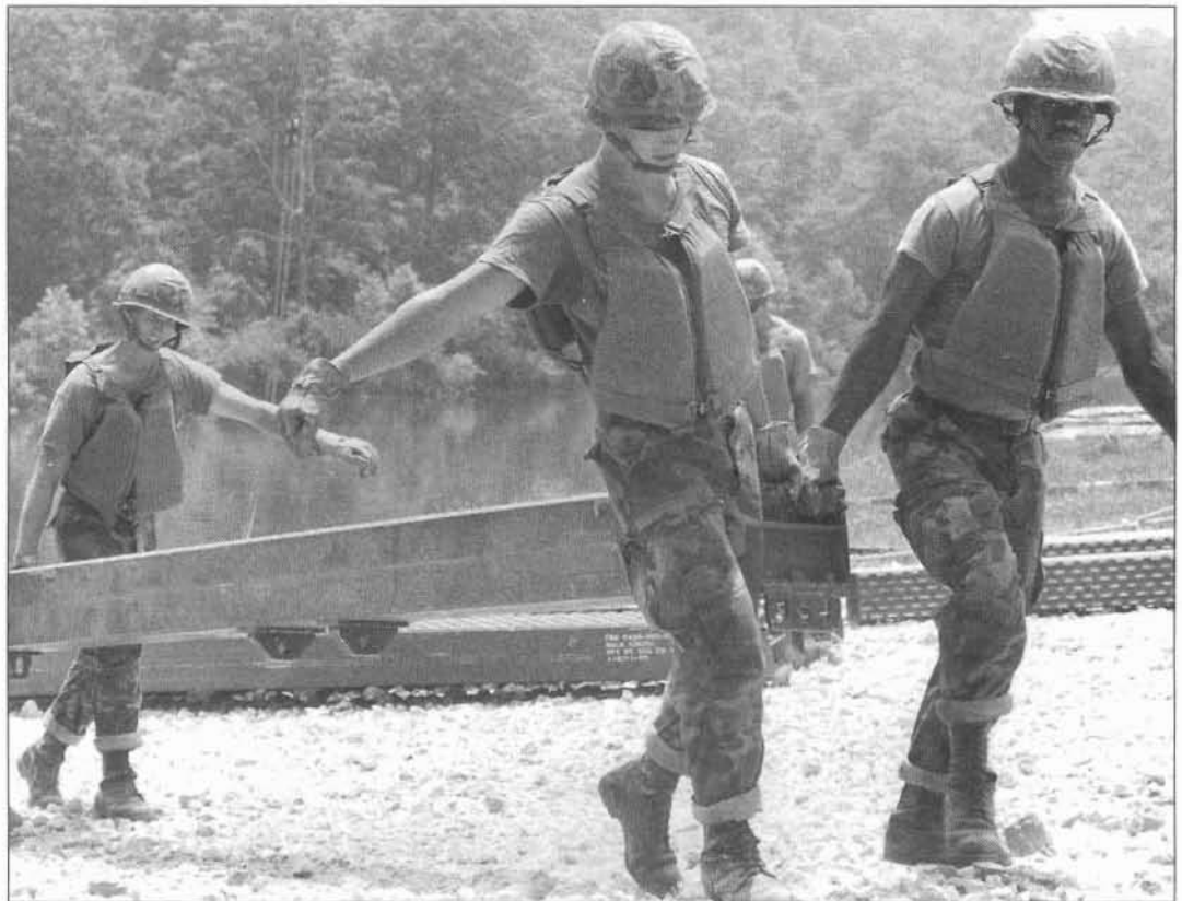
Engineers haul M4T6 long balk, which is used by Engineers as decking on fixed or float bridging. (Photo by SFC Dennis O. Lindsey.)
