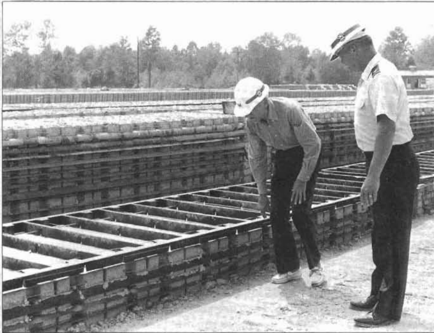
COL Dennis J. York explains construction of articulated concrete mats to Jacques Cousteau at the Delta Mat Casting Field. (Photo by Gary Dill.)
