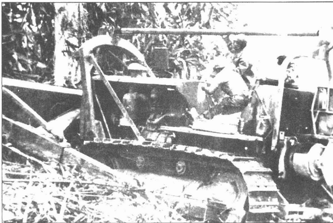
Engineers of the AFP clearing thick jungle for a road.
