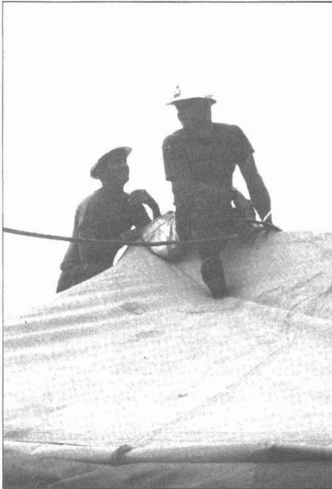
Engineers set up GP medium tents as temporary shelters for hurricane victims in South Florida.
