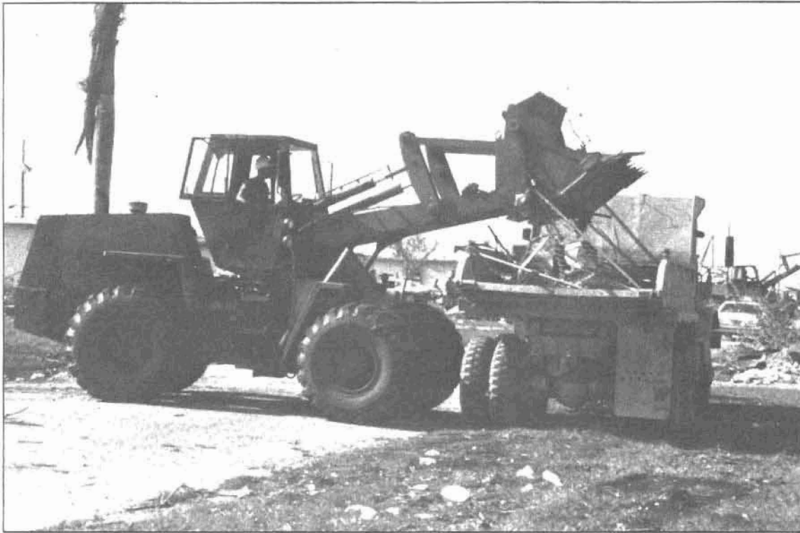
The 43rd uses a bucket loader to scoop up the enormous amount of debris left by Hurricane Andrew.
