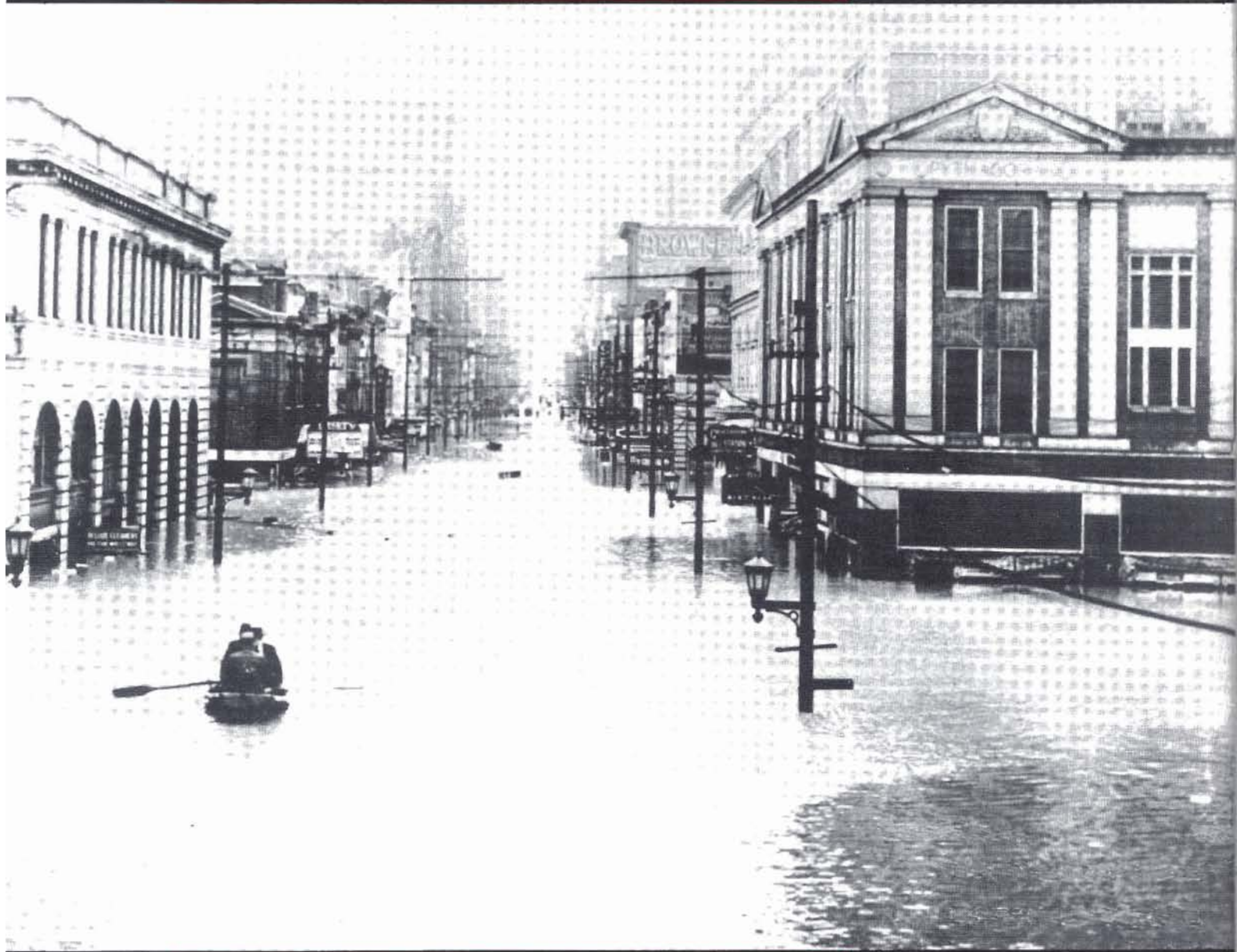
Wheeling, West Virginia flood conditions, March 18-19, 1936.
