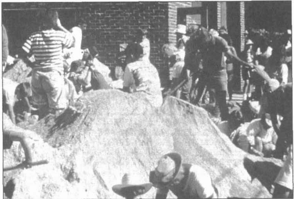
Volunteers fill sandbags at Roshenport, Missouri. The Corps provided more than 31 million sandbags to the midwest to hold back flood waters.
