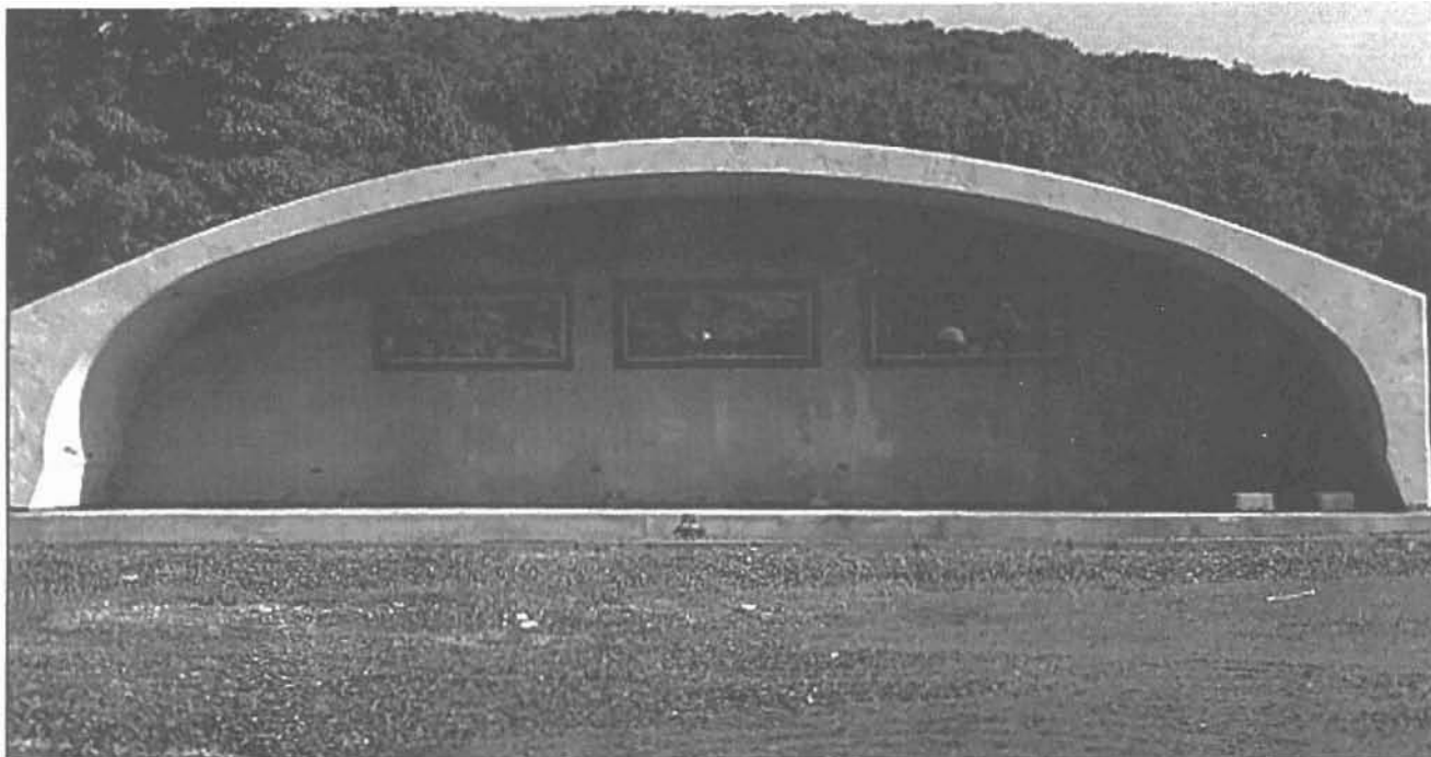
A completed bunker built with precast concrete.
