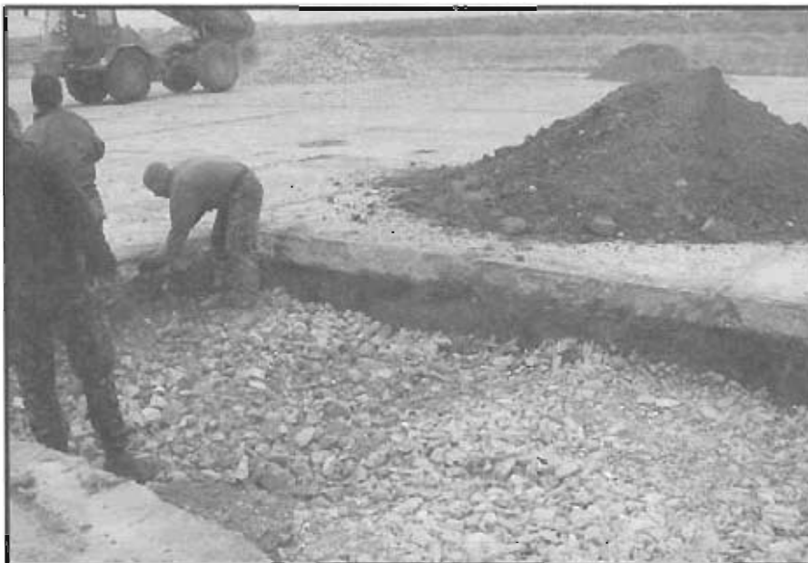
Soldiers perform runway repair work at Baghram airfield in Afghanistan.
