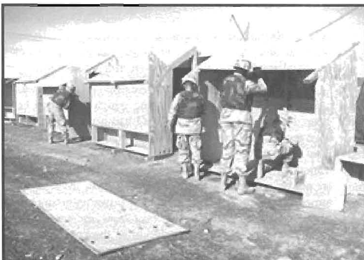
Engineer soldiers build latrines.
