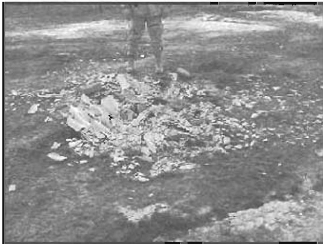
Damaged asbestos roof tiles present an environmental hazard.
