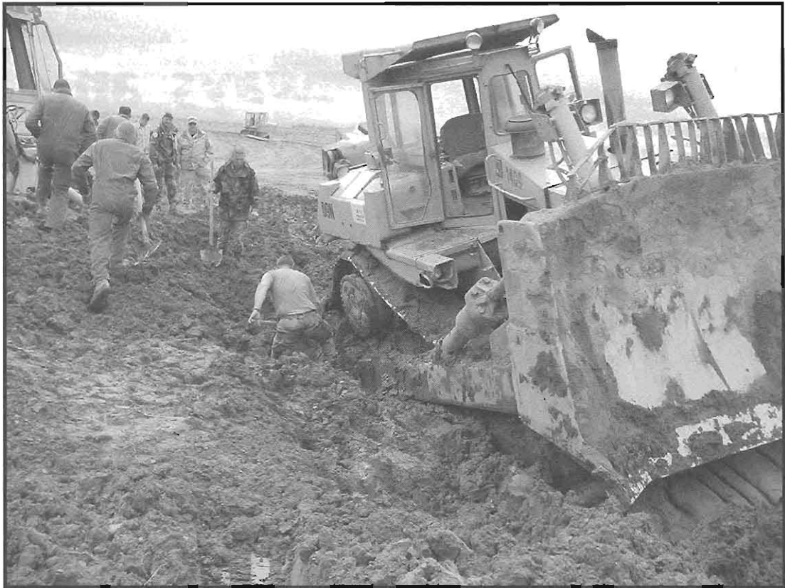
A dozer operates in difficult Central Asian terrain.
