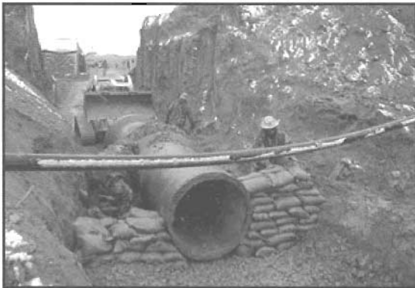
Engineers construct a head wall.
