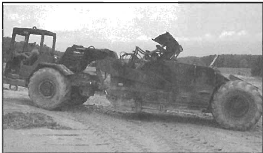
A scraper performs cut and fill operations.
