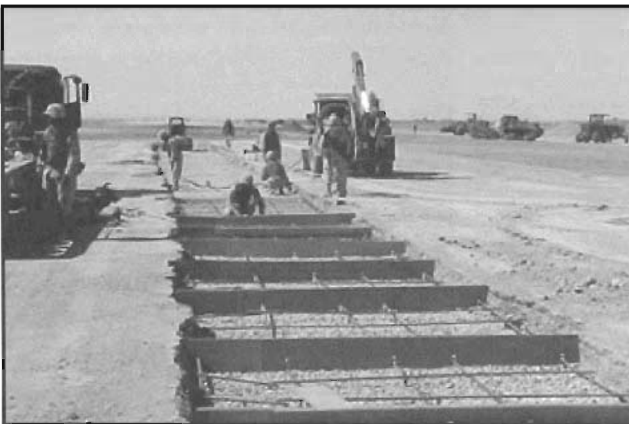
Engineer soldiers place concrete to repair a runway.
