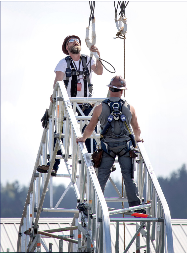
Two Shop 64 shipwrights use fall protection while working on a job near Dry Dock 3, April 24. (PSNS & IMF photo by Scott Hansen)
