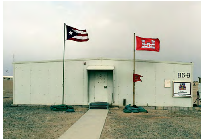
Building of the 215th EN CO Headquarters facilities in Kuwait. This is the starting point from where the unit "makes it happen" while mobilized in this mission. (Photo illustration provided by the 215th EN CO Vertical)
