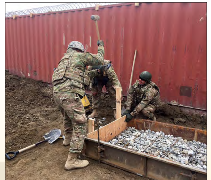
Members of the 215th EN CO (VER) prepare a mold for concrete pouring while deployed in Afghanistan. The main objective of this unit is the construction, remodeling, or demolition of facilities within their area of operations in the Middle East. (Photo provided by the 215th EN CO Vertical)
