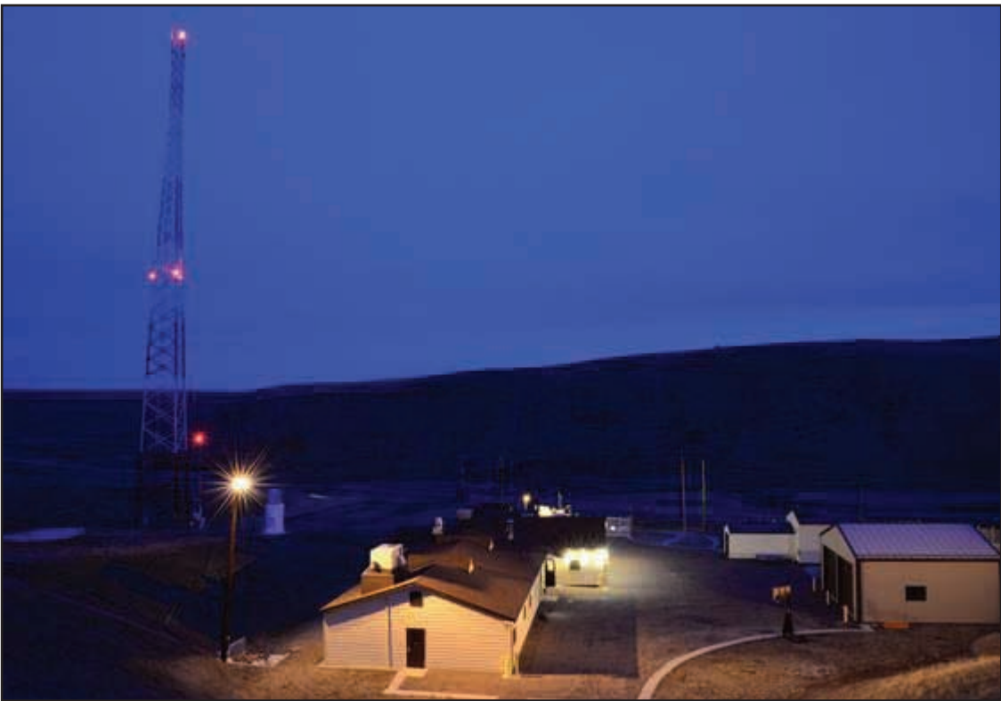
The sun begins to rise March 16, 2015, at a missile alert facility near Malmstrom Air Force Base, Mont. The M49 120 CFM gas filter, that recently passed a successful First Article Test at Pine Bluff Arsenal, is used in filter sets at MAFs. U.S. AIR FORCE PHOTO BY AIRMAN 1ST CLASS DILLON JOHNSTON (Taken from the Malmstrom Air Force webpage)
