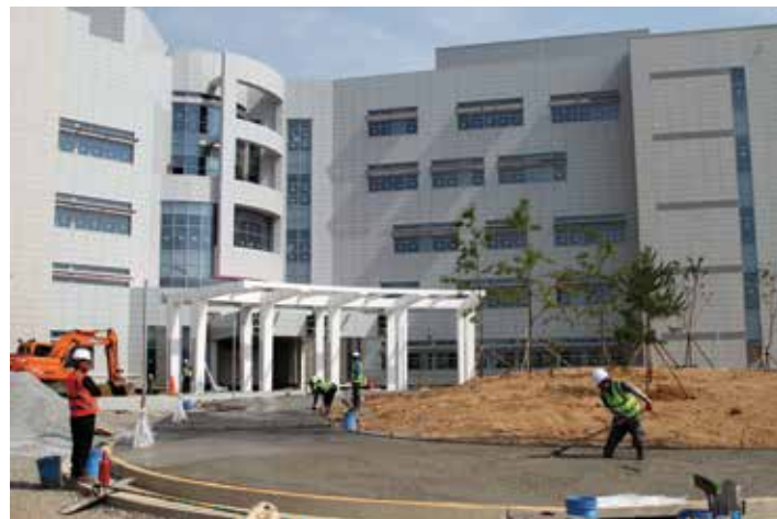
Current construction in progress
