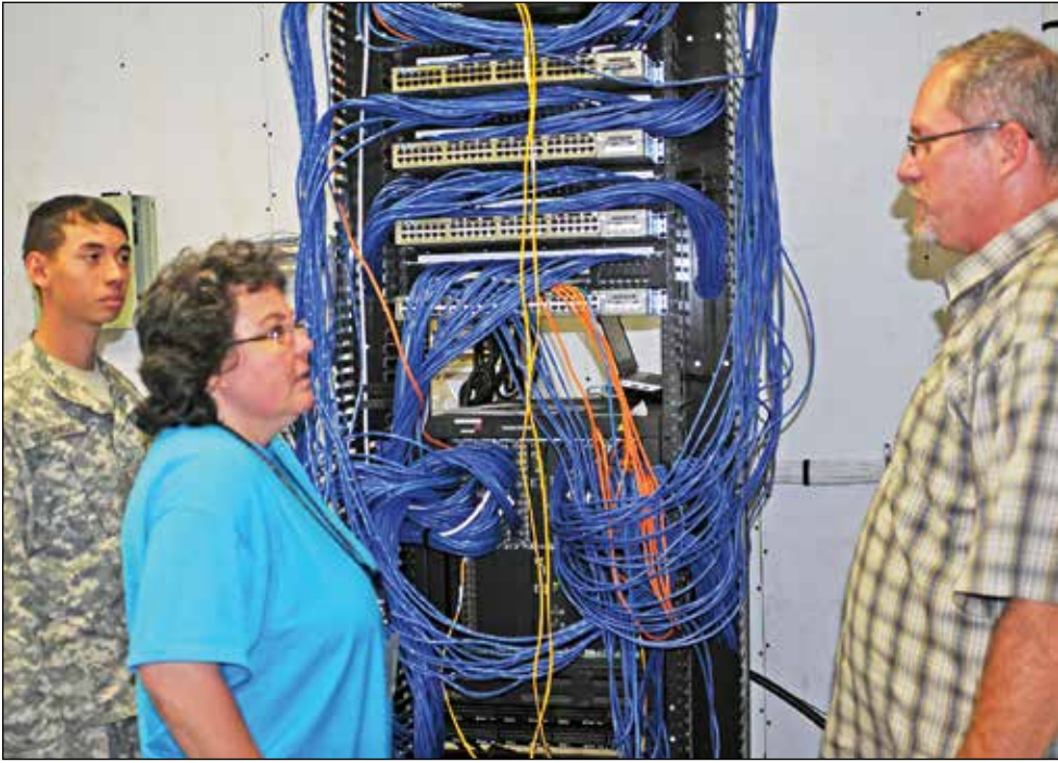
TOP: Pfc. Alan Rojas and Pfc. Everlidys Maldonado, both of Headquarters and Headquarters Company, 1st Sustainment Brigade, 1st Infantry Division, check specifications before continuing with their work replacing network switches and core routers at the headquarters of the 299th Brigade Support Battalion. MIDDLE: Spc. Jacob Reyna, 2nd Battalion, 34th Armor Regiment, 1st Armored Brigade Combat Team, 1st Infantry Division, loads a government vehicle with high-tech network components before heading out for a day's work. BOTTOM: Pvt. 2 Kenton Groombridge of the 1st Sustainment Brigade, 1st Infantry Division's S-6 shop, listens as Regional Network Enterprise Center project manager Julia Owens and RNEC technician Walter Moeller discuss a portion of the work needed to replace network switches and core routers at a Fort Riley military facility on Custer Hill.
