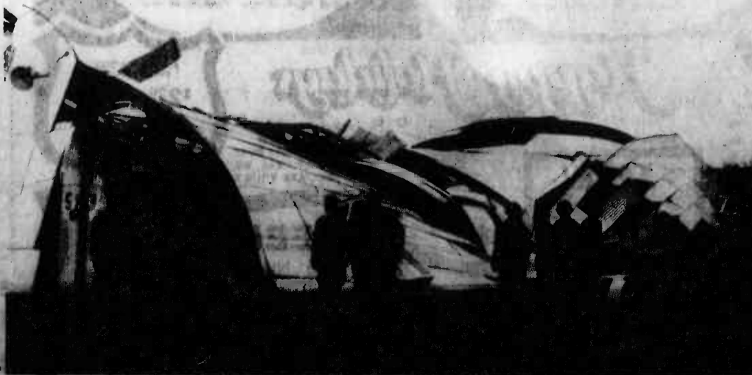
1st Radio Battalion's supply building completely collapsed during Hurricane Iwa. Marines survey wreckage, salvaging all equipment possible.
