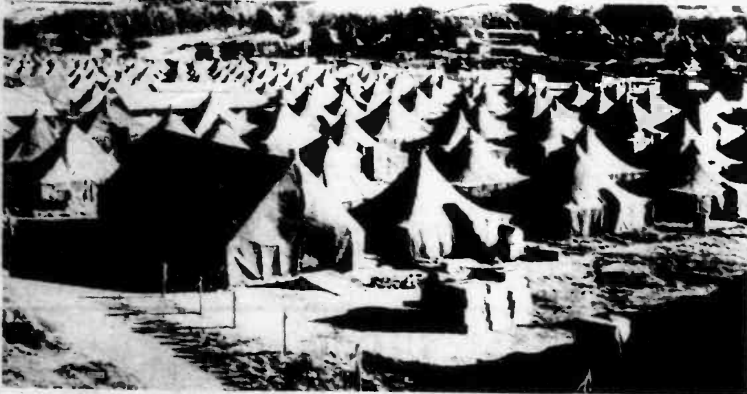
TENT CITY — Hundreds of tents sprung from the peaceful Kamuela countryside on the island of Hawaii in 1943 when the 2d Marine Division returned from their bloody victory at Tarawa. The large training base was called Camp Tarawa and
