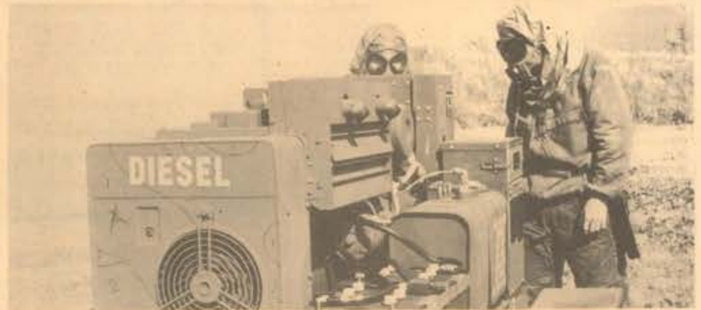
WHERE'S THE 'ON' SWITCH? — Maintenance personnel from Marine Air Control Squadron-2, attempt to start a diesel generator while clothed in Nuclear, Biological and Chemical protective gear. Routine maintenance was performed while "dressed out" in the NBC ensemble.
