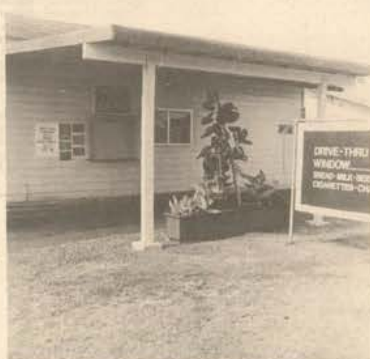
CLOSED PERMANENTLY — The drive-through window at the 7-Day store closed Sept. 18 due to the lack of business. The window is also considered a safety hazard for children playing in the housing area, according to an exchange official. (Photo by SSgt W.S. Saunders)
