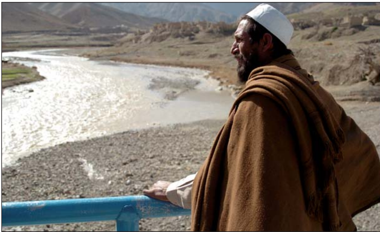
A local Afghan takes in the view from the newly-constructed Gogamanda Bridge in Kohe Safi.
